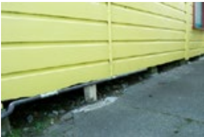
Figure 7: Areas of subfloor space with insufficient clearance
