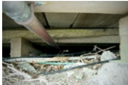
Figure 8: Areas of subfloor space with insufficient clearance
