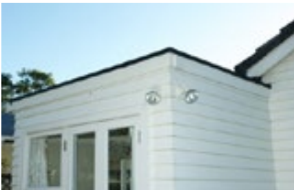
Figure 4: Bitumen membrane skillion roof
